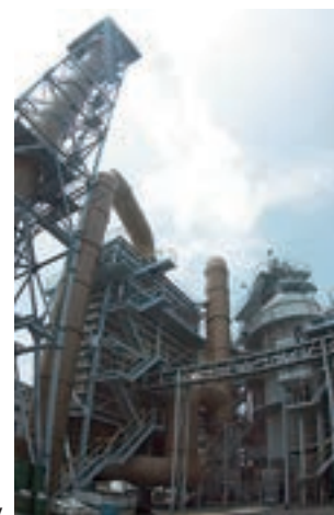
Industrial waste treatment facility
