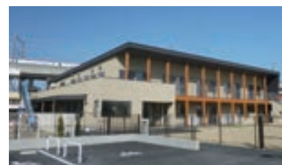
Construction of 'Sendai Nursery School' [Kurehanishiki Construction Co.]
