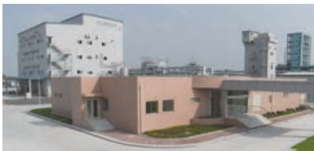
PVDF manufacturing plant in China
