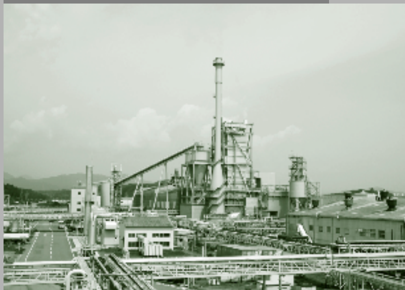
In-house power plant
