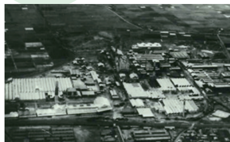
Kureha Chemical Industry Nishiki Plant
