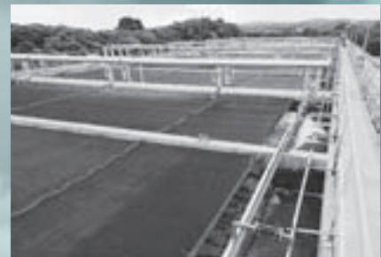
Wastewater treatment system
