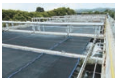
Wastewater treatment system
