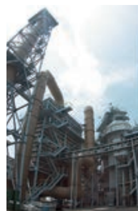
Industrial waste treatment facility
