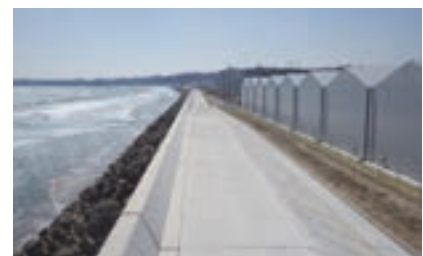
Reconstruction work completed for the Fukushima bay area [Kurehanishiki Construction Co.]
