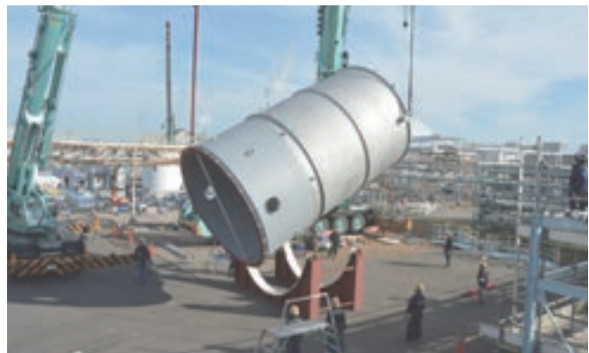
Construction is on-schedule
