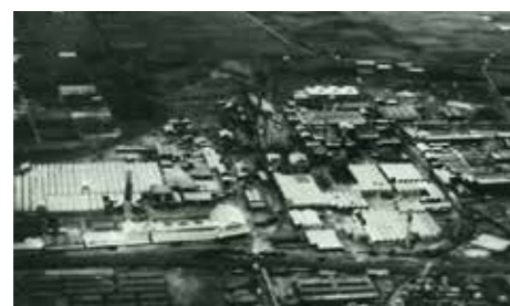
Kureha Chemical Industry Nishiki Plant
