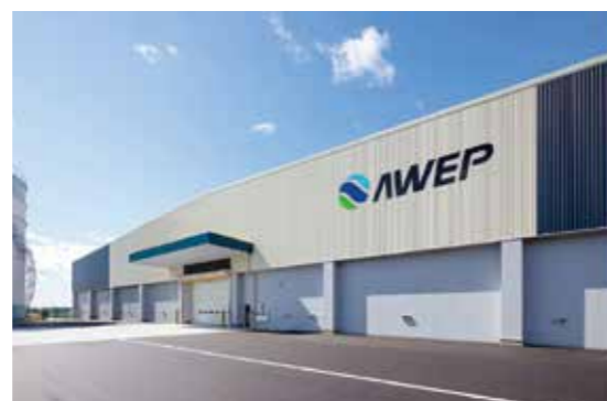
Kurehanishiki Construction Co., Ltd. FY2020 construction results: Wood pellet and PKS storage facility for AWEP Onahama Biomass Power Generation Project
